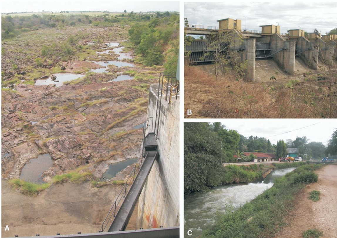
Figure S1. Photographic Evidence of the Reduced Discharge of the Walawe River and the Increased Discharge to the Catchment of the Other Rivers under Study (August 2004)
