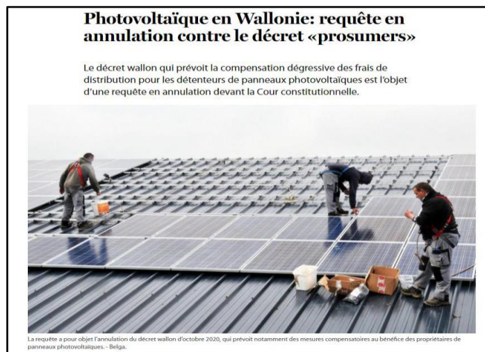
Figure 8: Pragmatic involvement in the energy system. Source: le Soir (2021)
