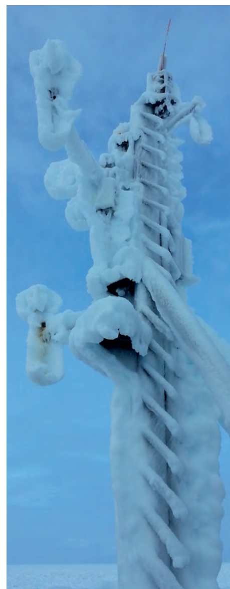
Figure 2: Despite the extra considerations for the Southern Ocean this ice storm took our system down for several months.
