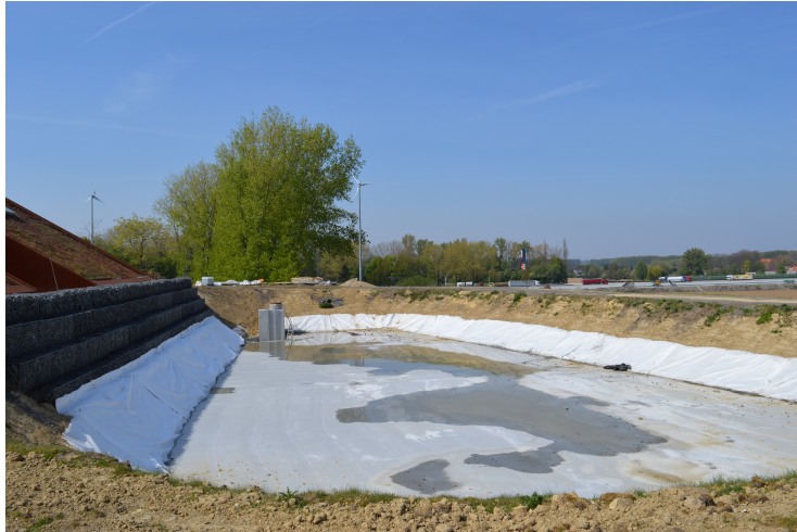
Figure 4.4: View of the upper reservoir in Quartier Negundo .
