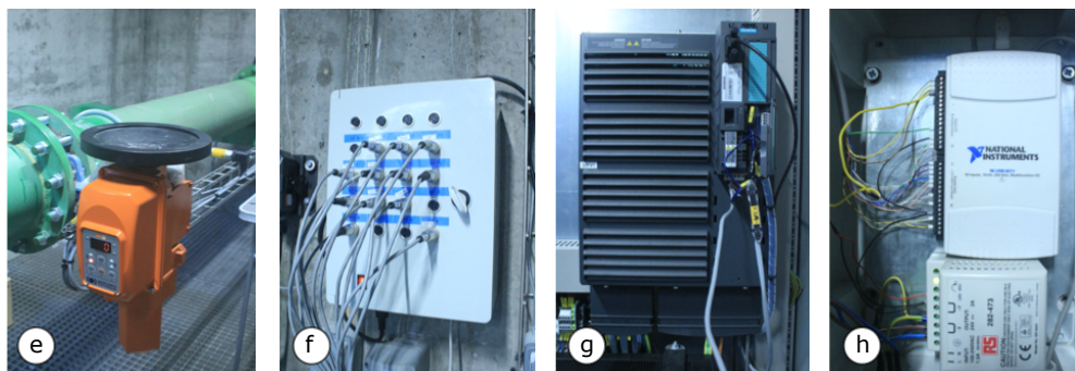
Figure 4.16: (e) electromechanical valve; (f) shunt box and connectors; (g) frequency driver; (h) acquisition card and sensors' electric tension supply.
