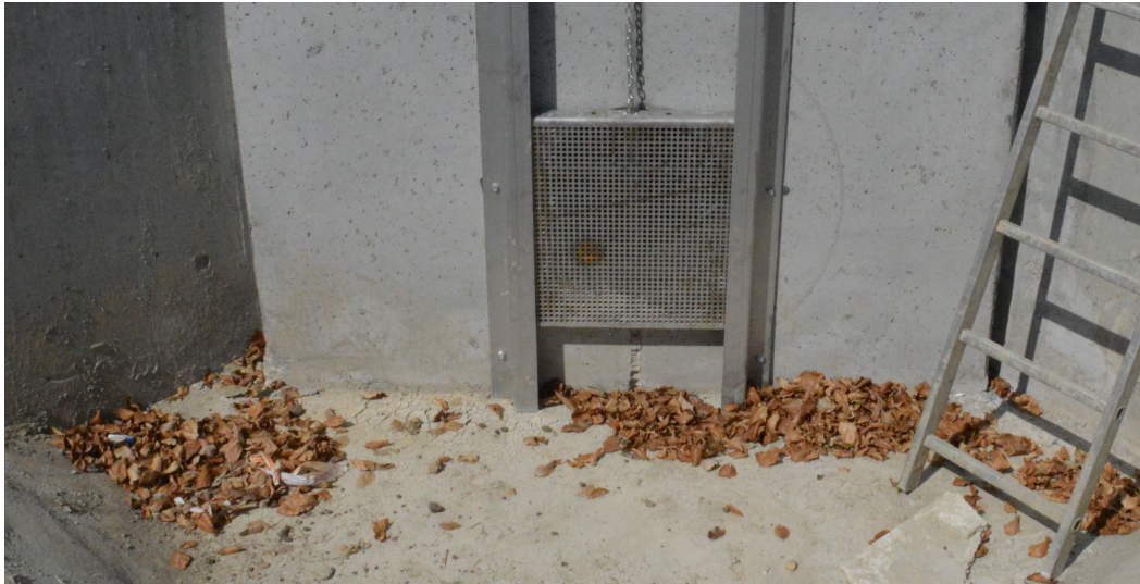
Figure 4.7: Photo of the trashrack cleaner at the upper reservoir pipeline inlet installed to protect the hydraulic system. The grid is removable for easing the periodic cleaning and maintenance. A similar grid is installed at the pump suction side.
