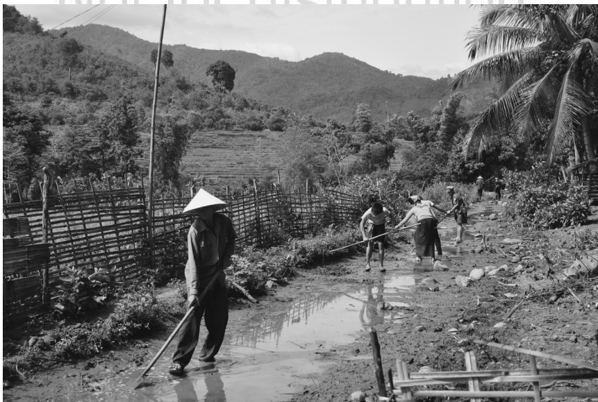
Figure 1.1 The maintenance of the lower canal (June 2010).
