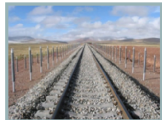
Figure 1.11: When strategic structure is built in not-optimal environmental condition, HPs are used to cool down the basement of the structure to avoid soil collapses.
