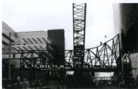
Figure 7.2: A truss pedestrian bridge at the Devos Hospital in Grand Rapids, MI, USA, undergoing construction. The loading of the bridge throughout its lifetime is subject to a large amount of random variation. Image courtesy of John Eisenschenk
