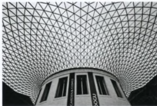
Figure 3.2: Grid shell roof structure by Buro Happold at the British Museum, London, UK. Image courtesy of Travis Simon
