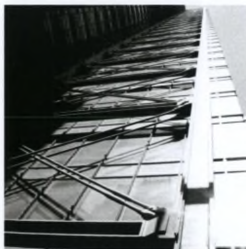
Figure 4.1: Bracing of the façade of a tall building, New York NY, USA. Image courtesy of Lionel Ponce
