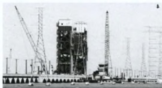
Figure 2.1: Numerous truss structures at the New Galveston Causeway Railroad Lift Bridge. Image courtesy of Patrick Feller
