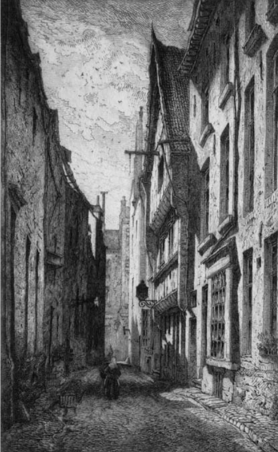
Fig. 2 – Corbelled wood façade in the Rue des Pierres. Engraving by Emile Puttaert, 1878 (© Archives of the City of Brussels)
