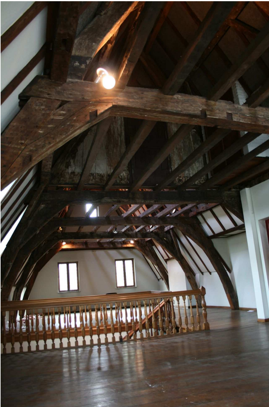
Fig. 4 – Roof frame of the house Brueghel, Rue Haute, no. 132 (© CReA-Patrimoine, ULB)
