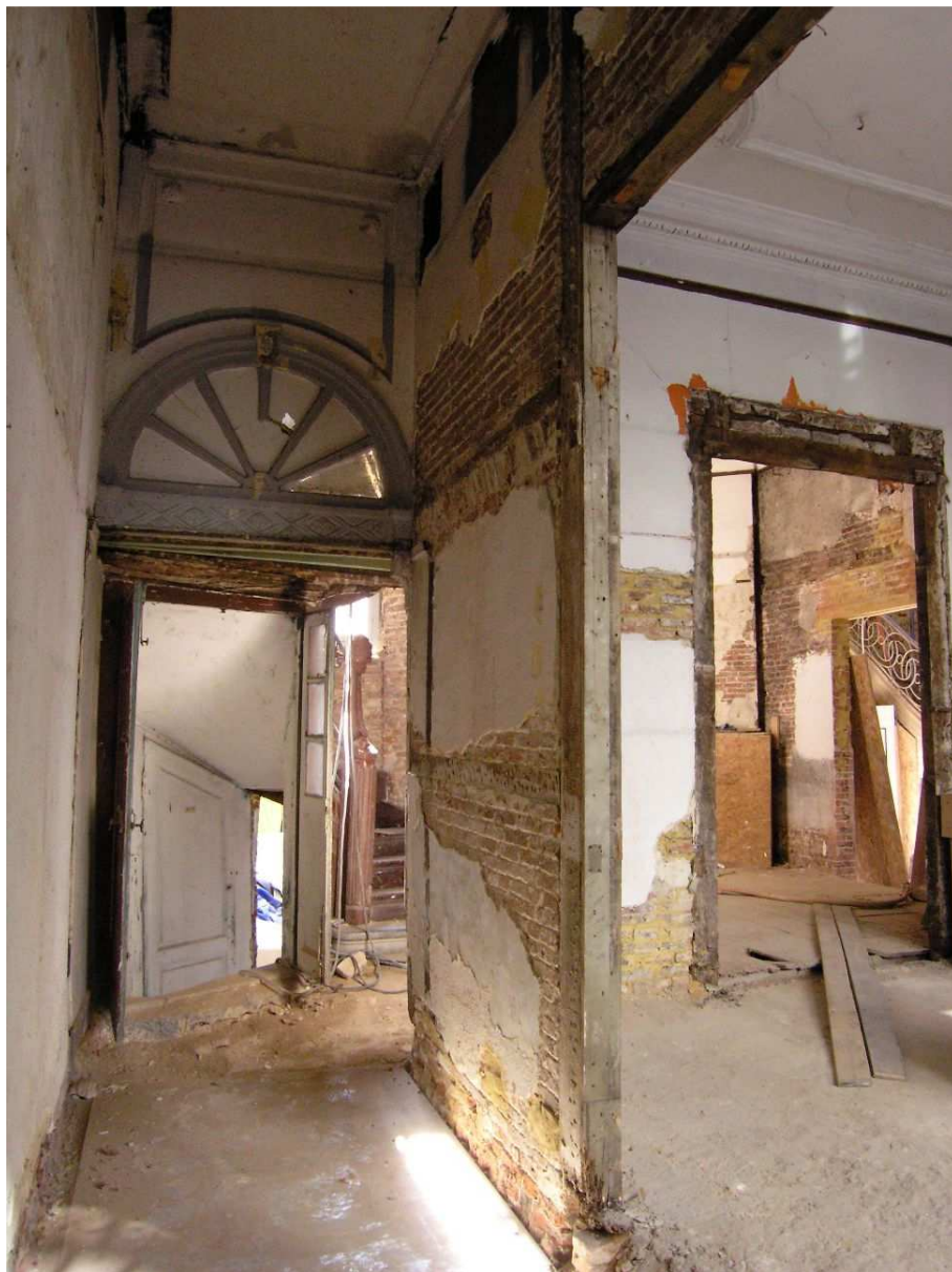
Fig. 10 – Timber-framed structure in the Dewez house, Rue de Laeken, no. 72-75, dated from the period 1789-1799 (© Royal Museum of Art and History, Brussels)
