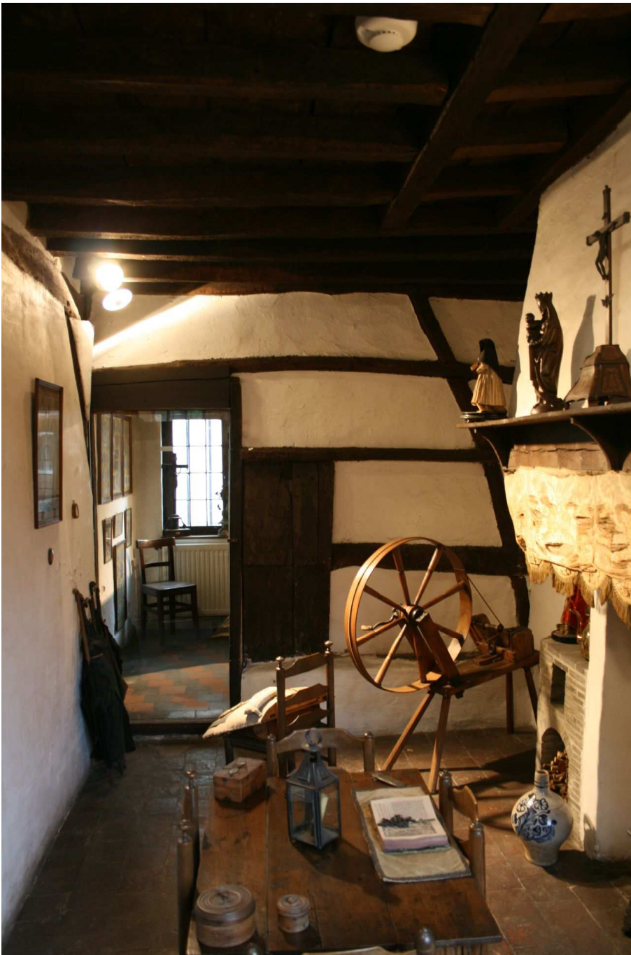
Fig. 8 – Ground floor of the Beguinage of Anderlecht. View of the timber frame dated from the first half of the 15 th (© CReA-Patrimoine, ULB)
