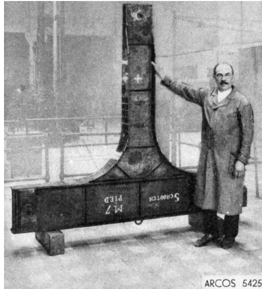
Fig. 2: Model of a node of the Schooten bridges for fatigue testing performed at the Université Libre de Bruxelles by Dustin (1935a).
